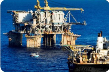
3R- 2 FPSO and 3R – 3 TLWP, now being upgraded
